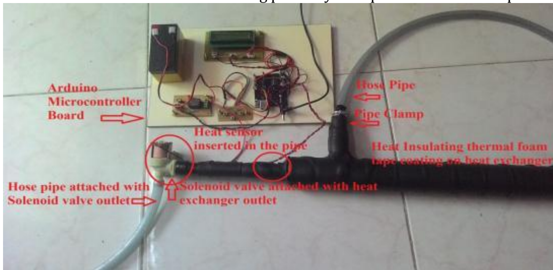
Figure 18: Arduino Microcontroller attached with the Heat exchanger
